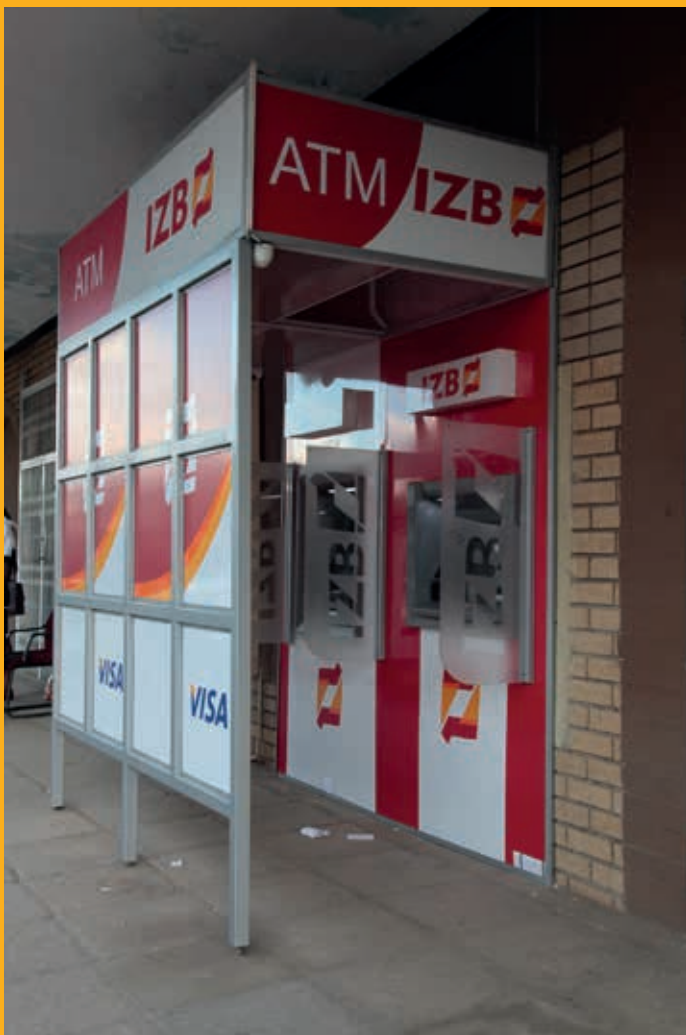
Cash recycler machine installed at the IZB Lusaka Main branch
